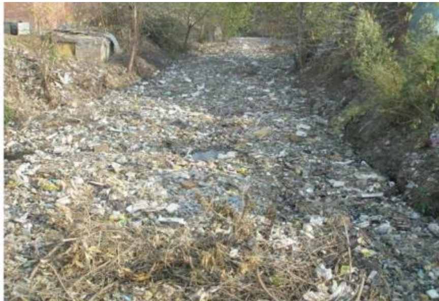
Fig. 8: Shadman drain carrying sewage and solid waste into the Ravi
